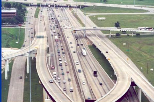
The Northwest Freeway also consists of 6 to 10 main lanes with 4 to 6 frontage road lanes. Current traffic on the Northwest freeway is more than 245,000 vehicles per day. It also includes a one-lane reversible, barrier separated HOT lane with 6 entry and exit points.
